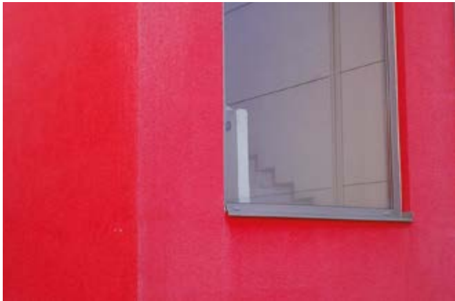
Colour fading due to an incorrectly selected shade
